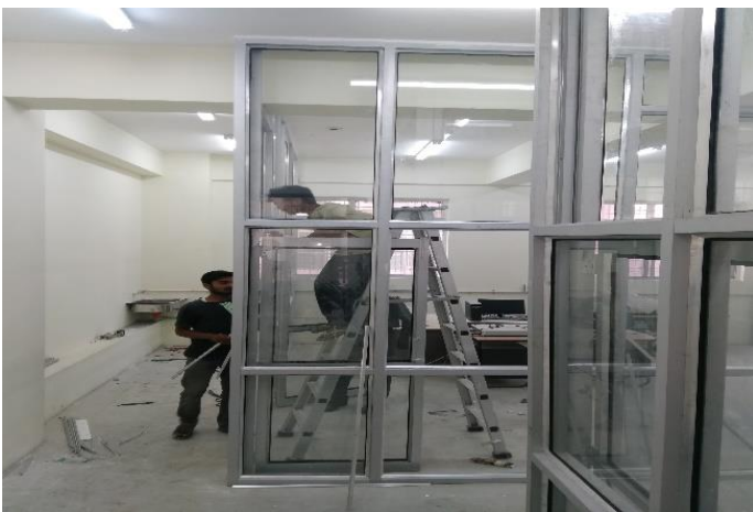
Al-Glass Cabin built as per need of different equipment, preparation of ramp for forklift move to carry out the high end research equipments.
